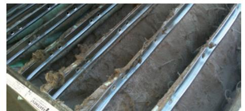
Vacuum machine filter at the conclusion of duct cleaning.
